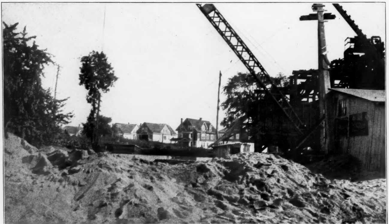
Derrick With Sand Pile in Foreground
